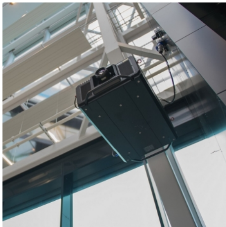
Panasonic PT-RZ31K laser projector in the vestibule
