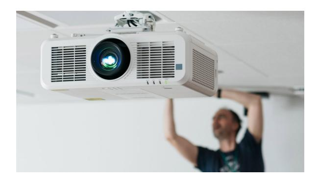
The six Group Rooms are equipped with a Panasonic PT-RZ570 laser 1-Chip DLP projector. With high brightness of 5400 lumens and excellent WUXGA image resolution and quality, with a 20,000:1 contrast ratio, it's an ideal solution for educational environments. The 360 degree installation option and up to 20,000 hours of maintenance-free operation, provide a highly flexible and reliable device.
