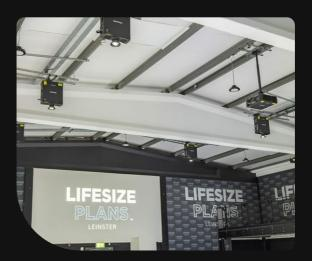
Panasonic's PT-RZ990 projectors provide 20,000 hours of maintenance-free operation, with lasting brightness and colour uniformity. The PT-RZ990 series of projectors feature a hermetically sealed optical engine and heat-pump based filter-less cooling design. This keeps projectors at the optimum temperature, and prevents dust ingress, especially when objects are being positioned on the showroom floor, to accompany the projection.
