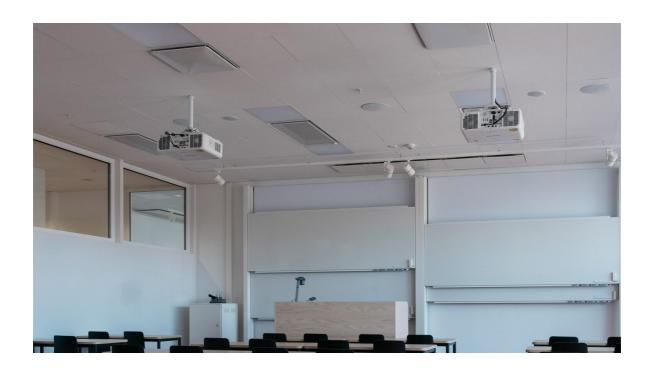
In total, there are 40 Panasonic projectors and 7 remote cameras for lecture capture and live streaming installed across the facility.
