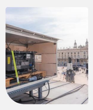
The projectors are all connected via single-mode fiber to the servers located in the basement of the town hall. The integration of cables is also discreet and buried under the cobblestones of the square.
